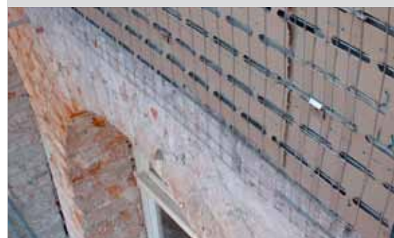
Bekaert Stucanet® applied in a facade renovation project with exterior plasterwork.
