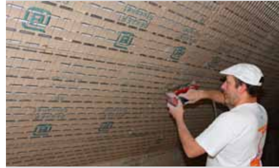
Quick and easy installation of Bekaert Stucanet® on wooden beams.
