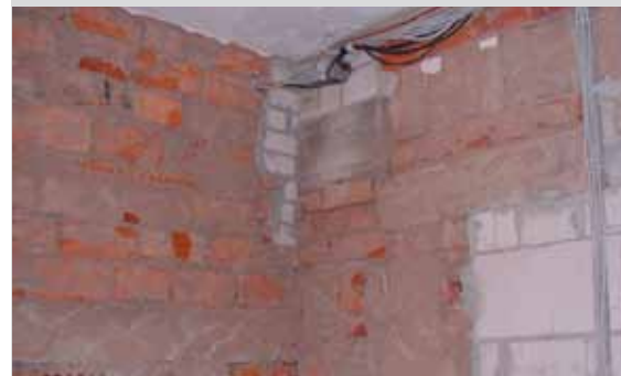
The substrate in renovation projects often consists of a mix of different building materials. Bekaert Stucanet® allows the durable renovation and plastering of this type of difficult walls.
